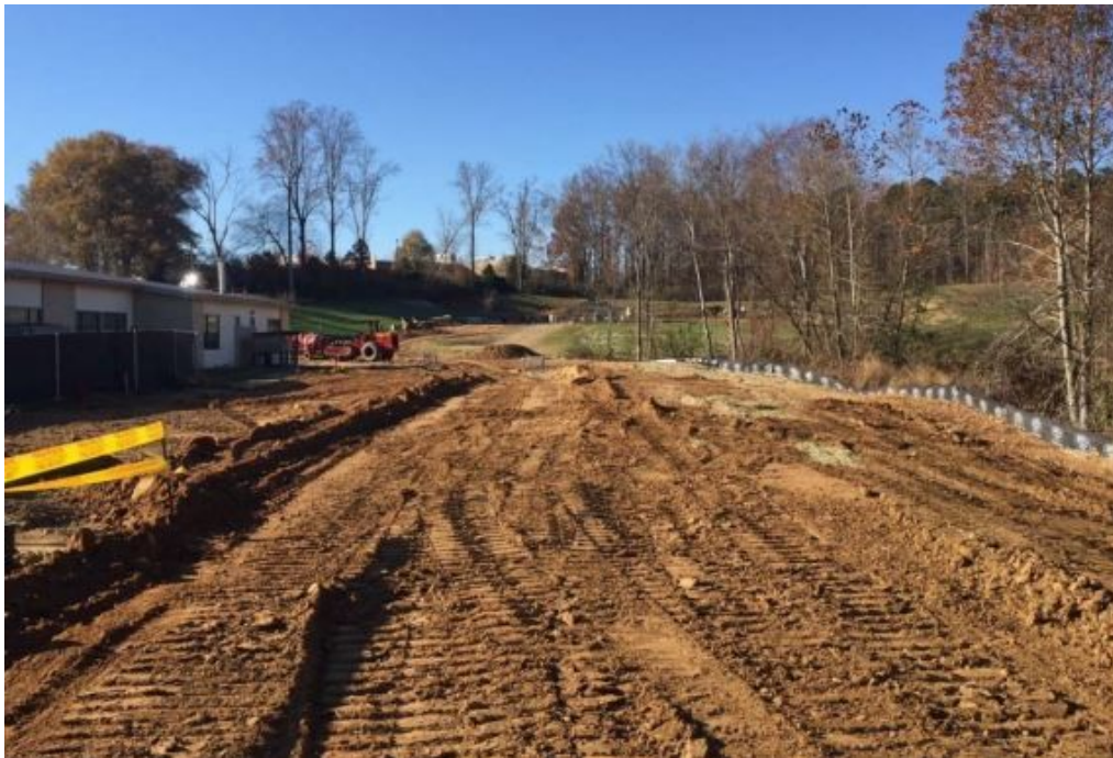
View of rear emergency vehicle road
