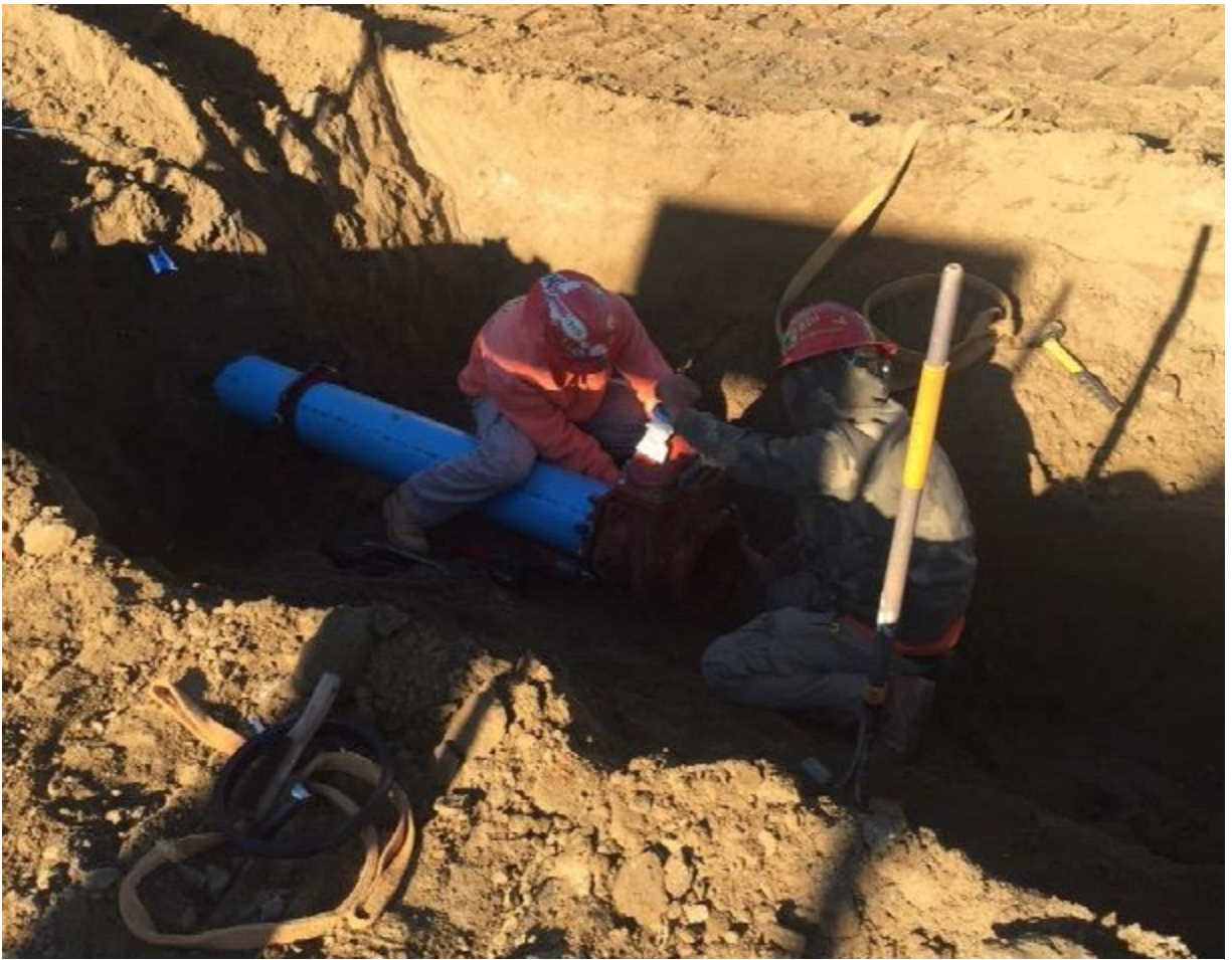
New utilities being re-routed and connected
